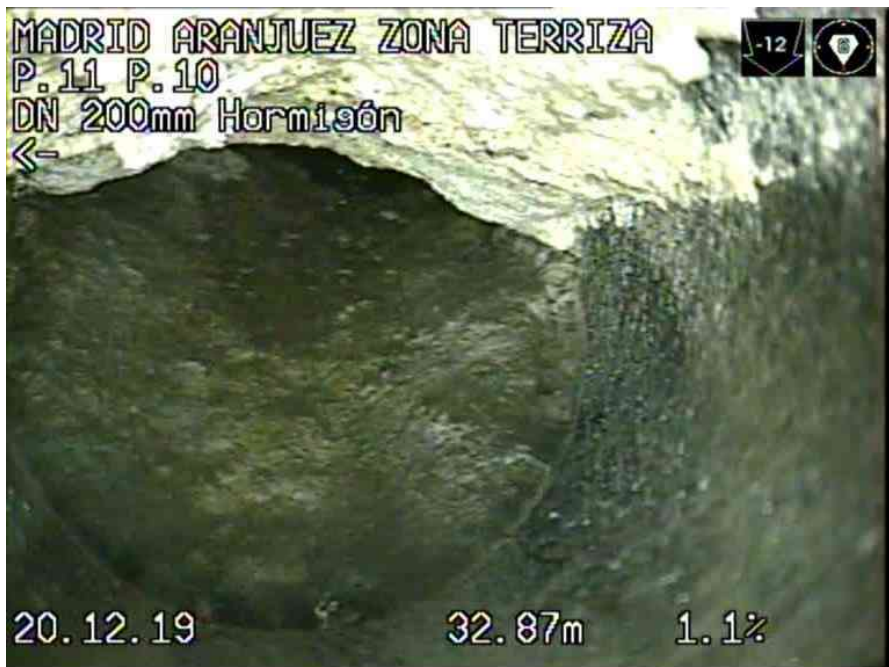
1_6615eaf7-0e8f-43b5-8cc1-c3c7e07ff22d_20191220_122036_071.jpg, 00:03:48, 32.73 TUBERÍA HUNDIDA
