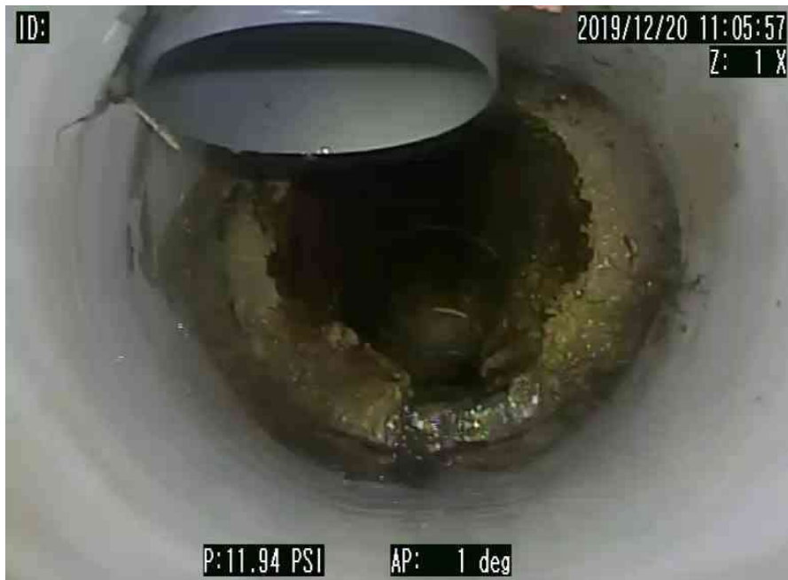
3_67b9b3b9-a48f-443e-b804-f41a69aa9dc8_20191220_122702_363.jpg, 00:00:00, 15.00 FINAL DE LA INSPECCION
