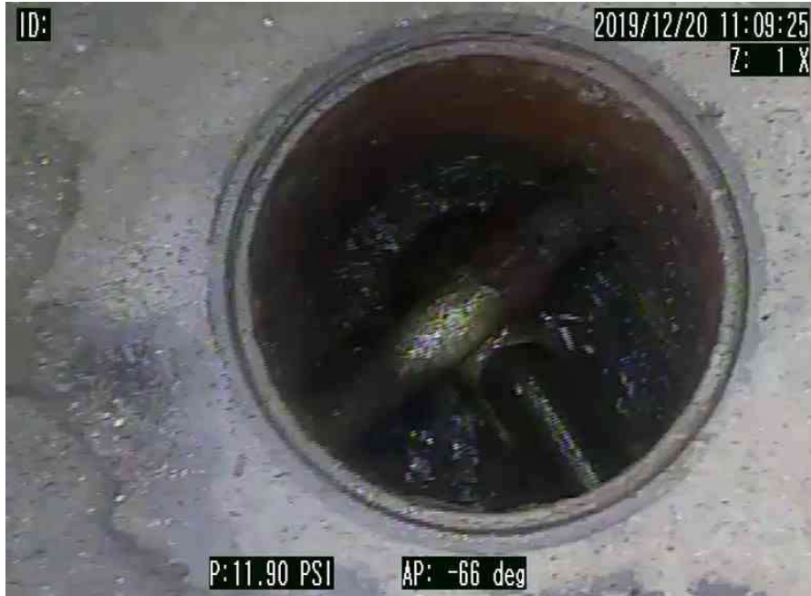
3_8a41291f-fc46-40b1-9441-dec0f23b898f_20191220_122652_509.jpg, 00:00:00, 0.00 INICIO DE LA INSPECCION
