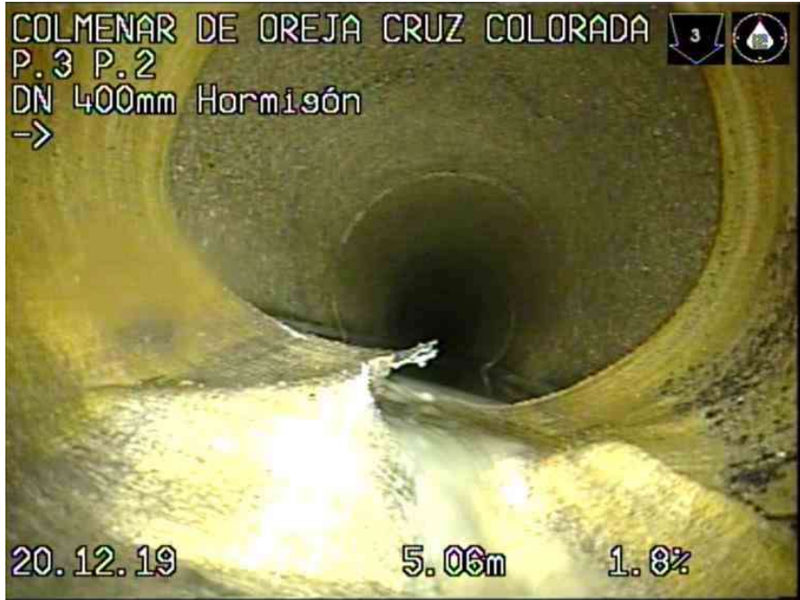
5_fd54914d-5f58-41d6-8e02-7be684dc4f05_20191220_091749_380.jpg, 00:01:16, 5.06 FINAL DE LA INSPECCION
