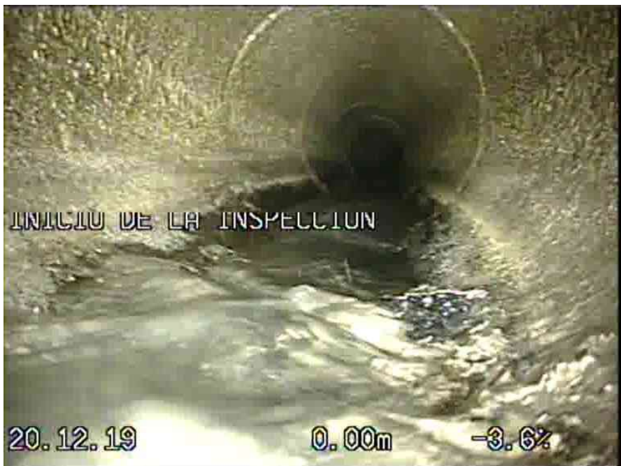
2_e1fb489d-1487-41a9-988d-93f77cca59c9_20191220_083446_362.jpg, 00:00:04, 0.00 INICIO DE LA INSPECCION
