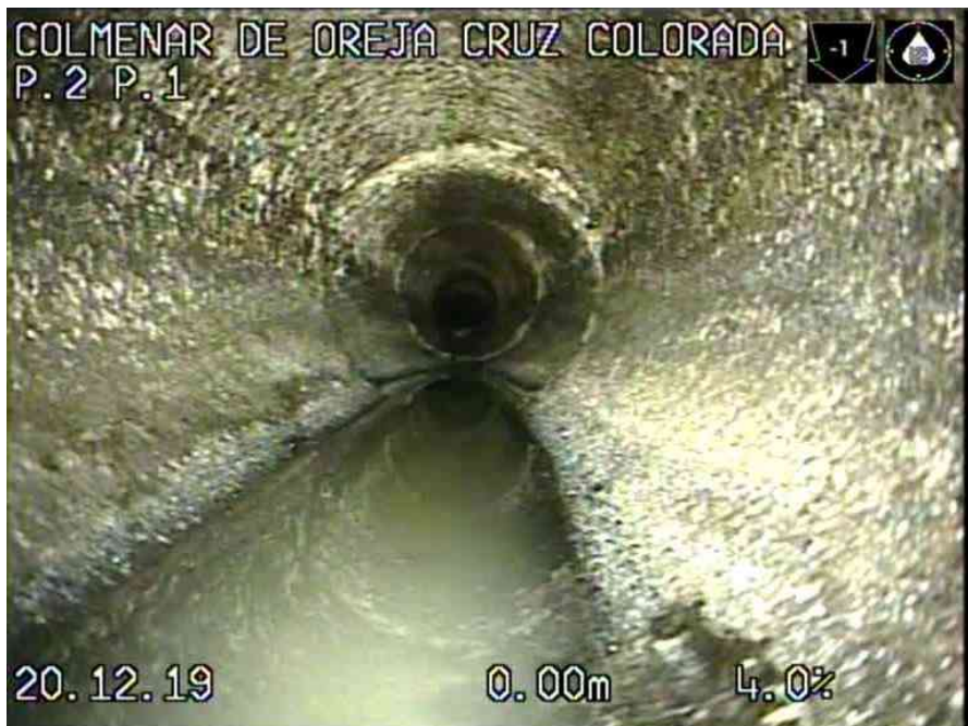
1_22d328f5-3deb-4699-9e14-0280fc7809e9_20191220_082853_854.jpg, 00:00:03, 0.00 INICIO DE LA INSPECCION
