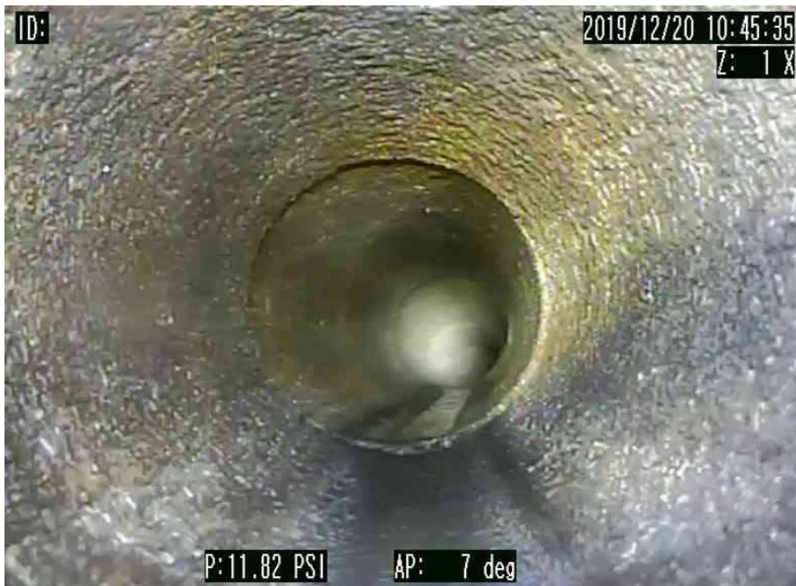
7_5f64e322-e94c-4f37-8634-834cc01d3561_20200102_175342_050.jpg, 00:00:00, 13.20 FINAL DE LA INSPECCION
