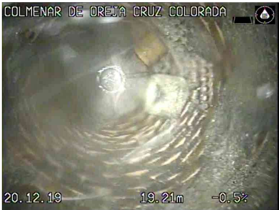
3_592609d1-4a32-4db8-981c-bad4889cf6fa_20191220_092256_109.jpg, 00:02:30, 19.21 FINAL DE LA INSPECCION
