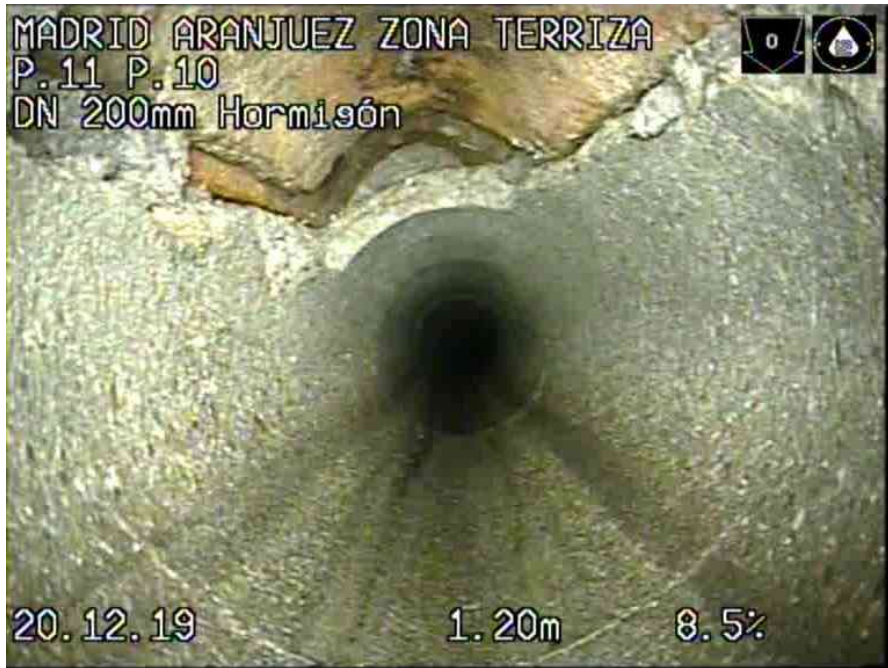
1_ed68046c-41a0-40bf-b4c6-91572264d1a2_20191220_121428_301.jpg, 00:00:01, 1.20 INICIO DE LA INSPECCION
