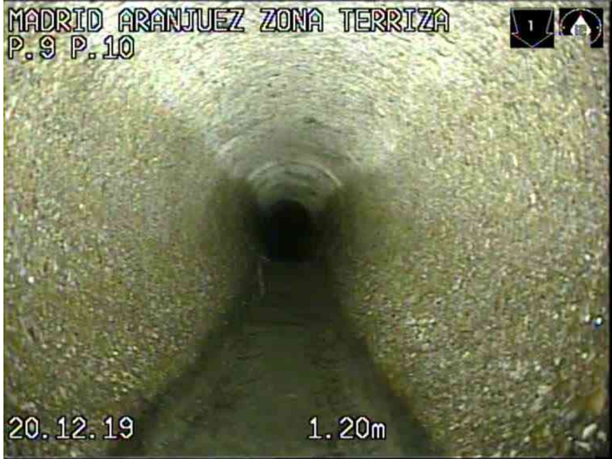
2_deaf2da5-aa69-43e4-9e78-81ce9a4aa3a5_20191220_123915_651.jpg, 00:00:01, 1.20 INICIO DE LA INSPECCION
