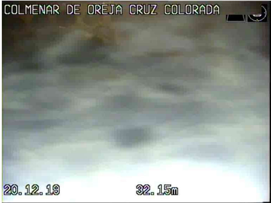
4_4030601e-2d56-43b9-8536-0f45bd24e705_20191220_092904_954.jpg, 00:03:46, 32.15 FINAL DE LA INSPECCION
