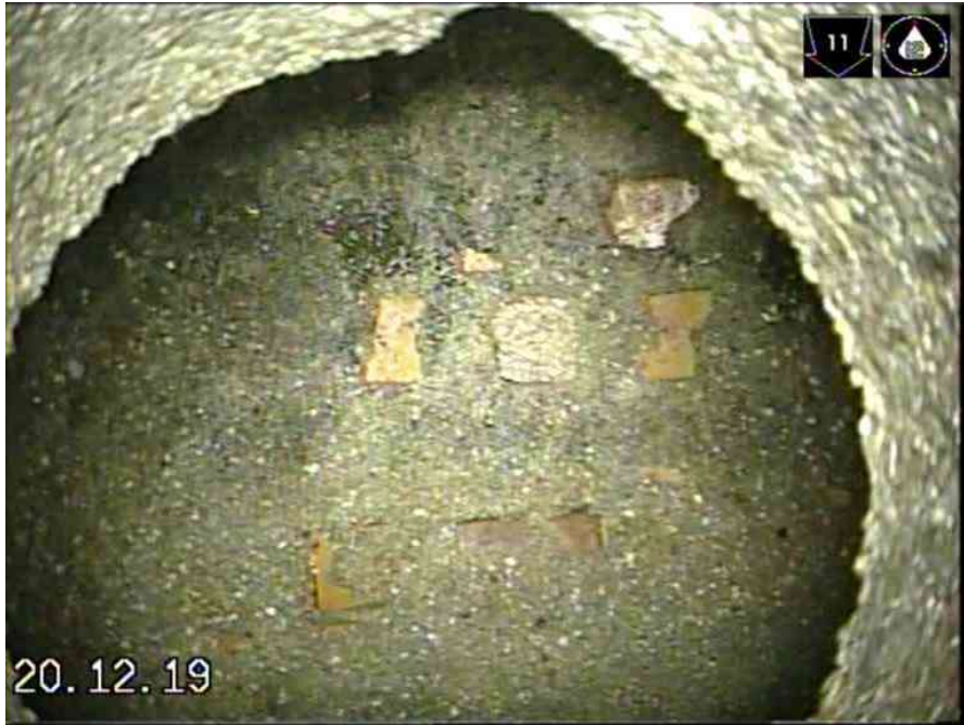
2_22a9b150-fee8-45d4-b4de-85375761b18f_20191220_124407_088.jpg, 00:04:09, 42.21 FINAL DE LA INSPECCION
