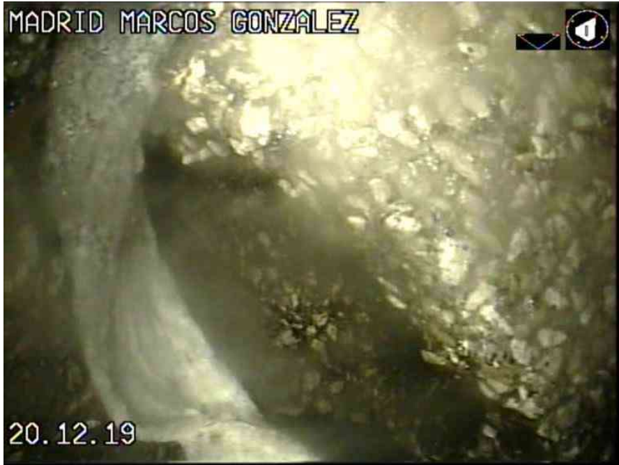
2_8e916f5d-c9b8-4dea-bc94-507324ae2ca7_20191220_113717_103.jpg, 00:01:29, 6.88 FINAL DE LA INSPECCION
