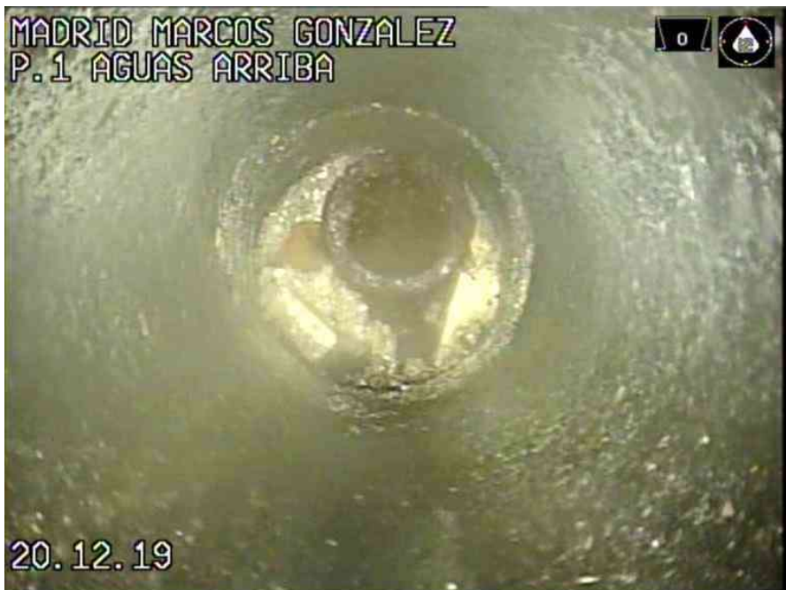
4_bb858c2c-c4c9-4474-82ea-f245c52340c8_20191220_114933_479.jpg, 00:02:31, 22.02 FINAL DE LA INSPECCION
