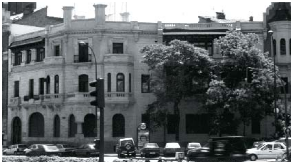
Vista general S
